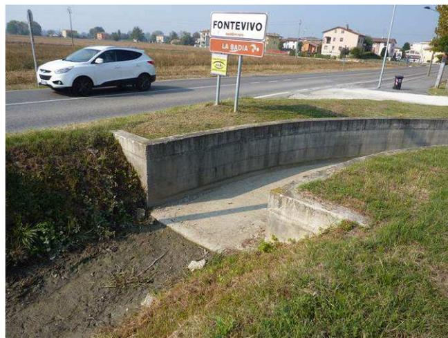
FIGURA 6-6 – CANALE NUOVO – SEZIONE AD "U" IN C.A.
