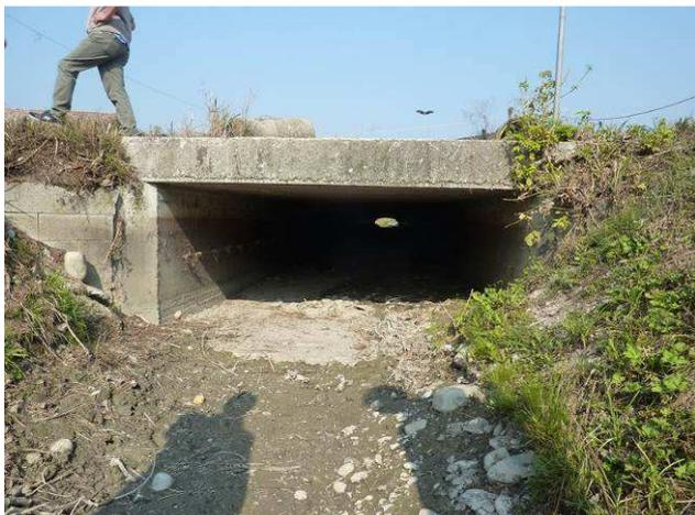
FIGURA 6-3 – CANALE NUOVO - IMBOCCO TOMBINO SCATOLARE IN C.A.
