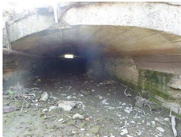
FIGURA 6-4 – CANALE NUOVO - SBOCCO TOMBINO AD ARCO IN MURATURA
